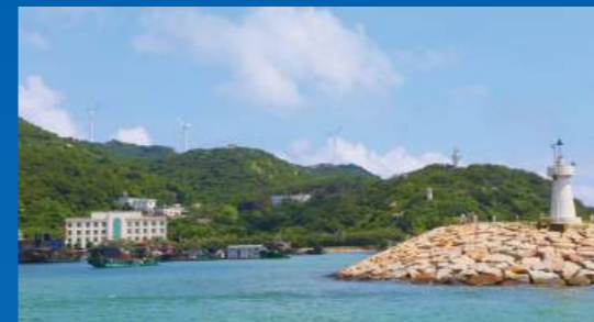
珠海东澳岛智能微网 Zhuhai Dongaodao Smart Microgrid
