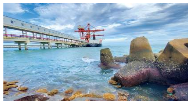
越南永新项目采用先进技术实现废水“零排放”，维护良好的生态环境，项目码头区域的珊瑚生态系统得到了蓬勃发展 The Vinh Tan 1 BOT Coal Fired Power Plant Project adopts advanced technology to achieve Zero Discharge of wastewater, preserving sound ecological environment. The coral reef ecosystem near the dock area of the project survived and thrived
