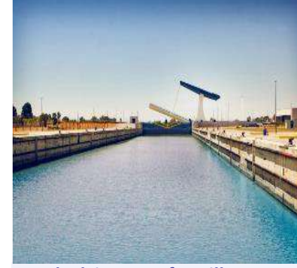
New lock in port of Seville, SPAIN
