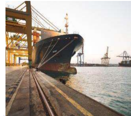
Extension and improvement of the public container terminal, Valencia, SPAIN
