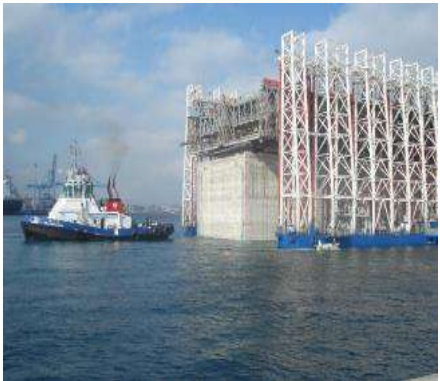
Construction of new breakwater and quay extension, Algeciras, SPAIN
