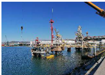
Extension of the existing jetty for loading LNG vessels up to 80,000 m 3 , Barcelona SPAIN
