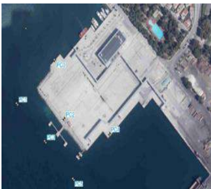
Port expansion, “Poniente” quay and yard, Alcudia, SPAIN
