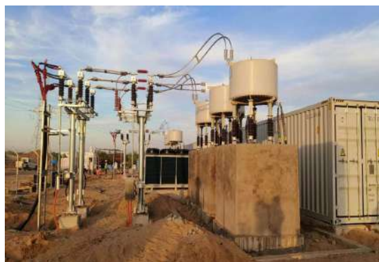
Renew 200MVar Wind Plant@Karnataka, TSVG-50/33-W-C
