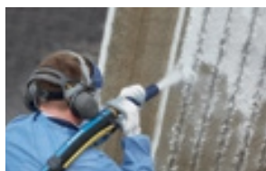
8.6 to 10 bar: Abrasive blasting
