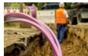
12 to 14 bar: Cable blowing and drilling
