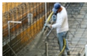
7 to 12 bar: Shotcrete applications
