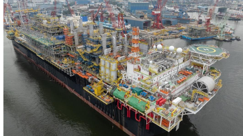
P78 FPSO SEATRIUM PETROBRAS - BRAZIL
