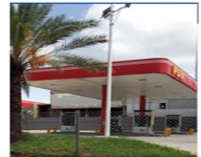
GNV PROJECT GLP PIPELINES CORPOVEN
