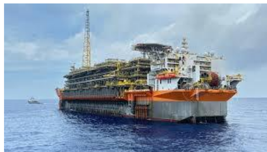
ALM. TAMANDARÉ FPSO SBM PETROBRAS - BRAZIL
