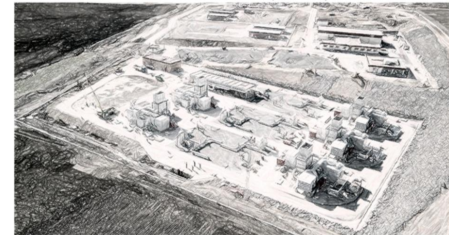
CABORCA COMPRESSION GAS CARSO BAJA CALIFORNIA - SONORA
