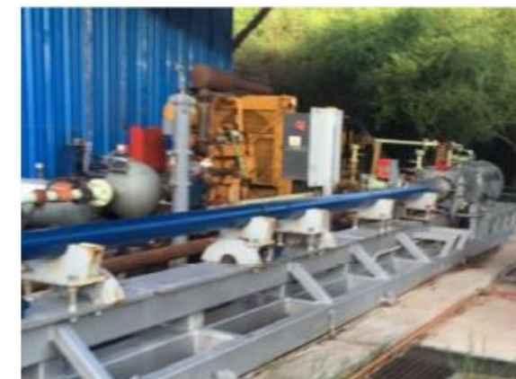
Customer: Ecopetrol, Castilla Field Project: Repair, Tests and Start UP 2 HPS 80,000BPD@1200PSI-2500HP
