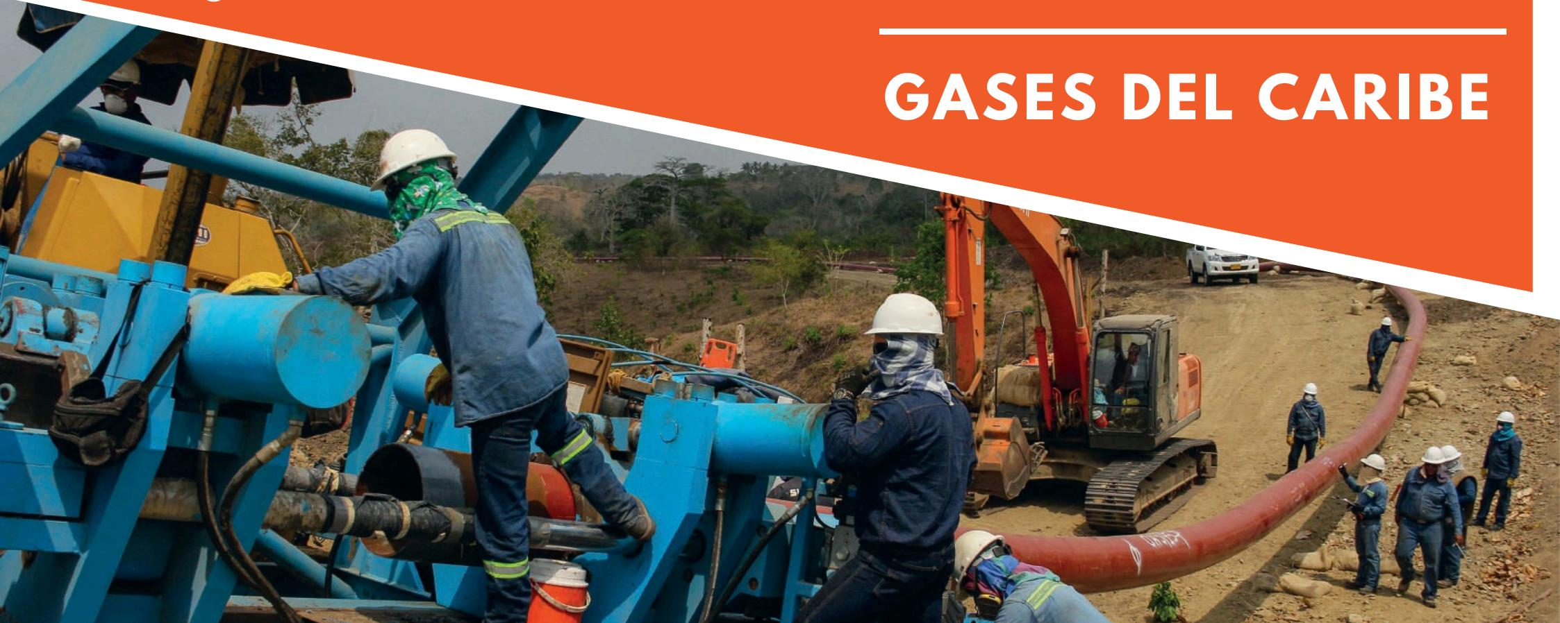
A photograph showing a construction site for a gas pipeline. In the foreground, a worker in a blue uniform and white hard hat is operating a large blue hydraulic machine, possibly a pipe cutter or alignment tool. Another worker is visible in the background near a red excavator. The site is in a hilly, dry landscape with other workers and equipment in the distance. A large red gas pipeline runs along the right side of the image.
